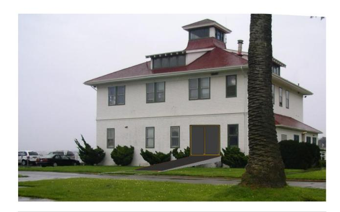
[7]: Proposed Boathouse Ramp (Building 1903): This ramp is an artist's rendering of a recreated ramp to the boathouse, in its pre-existing location that provides access to the re-constructed boathouse doorways. Colors of non-skid ramp surface, doors and trim to be submitted to GGNRA for review. (Photo and illustration by NPS staff, 2007.)
