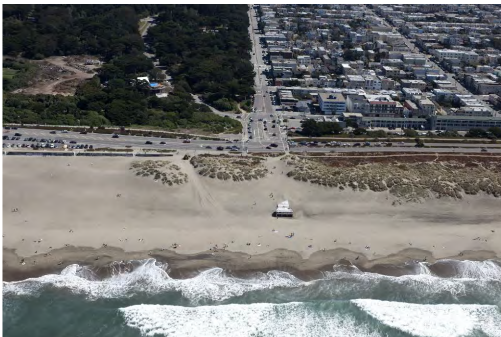
Figure 9: Outfall structure located along Ocean Beach.
